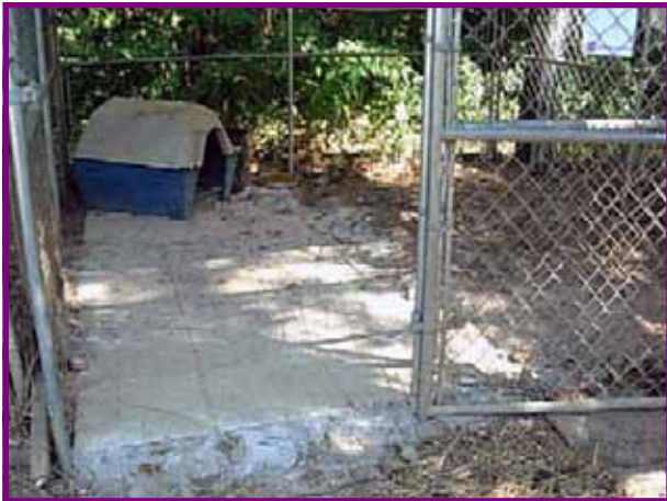
"Finished Product" One of the newly paved pens. Great job, everyone!
